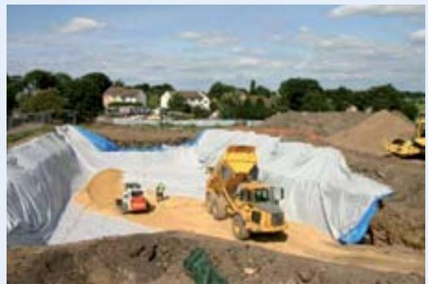
**Stage 4:** Protect the root barrier membrane from tyre damage with a layer of sand.
