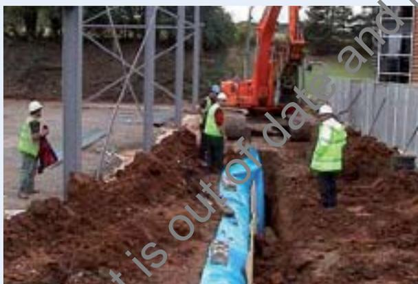
**Stage 3:** Support the root barrier membrane with shutters, pile and backfill the trench.
