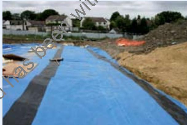
**Stage 8:** Protect the surface of the cell with sand and bury deep enough to prevent disruption in the future.
